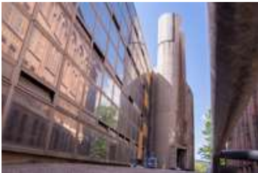
Photo 5. National Electric Power Distribution Station in Budapest (Hungary), designed by Csaba Virág in 1972—1974 that got demolished in 2020. Photo of Dorka Bartha (We Love Budapest)
