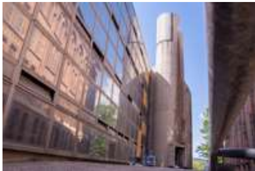
Photo 5. National Electric Power Distribution Station in Budapest (Hungary), designed by Csaba Virág in 1972—1974 that got demolished in 2020. Photo of Dorka Bartha (We Love Budapest)
