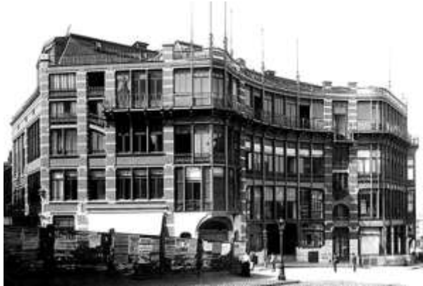
Photo 2. The former Maison du people (“House of the People”) in Brussels(Belgium), designed by Victor Horta (1896—1898) that was demolished in 1965 by the city’s authorities in spite of the protest of many architects and the international committee of the Venice Charter for urban development purposes (a skyscraper was built on its site).
